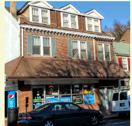
A historic structure in the City of Fredericksburg is retrofitted to provide a neighborhood commercial use and upper-story housing.
